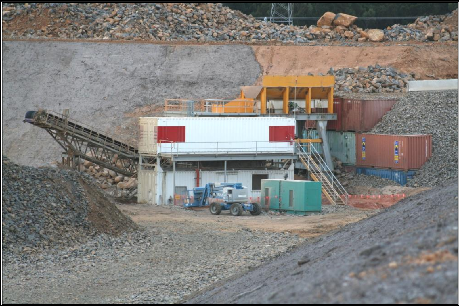
Rock crushing plant on the Longreach site.
