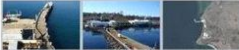
One of the fingers of the wharf. Freezer plant and fish meal factory at Aerial view of the wharf.
