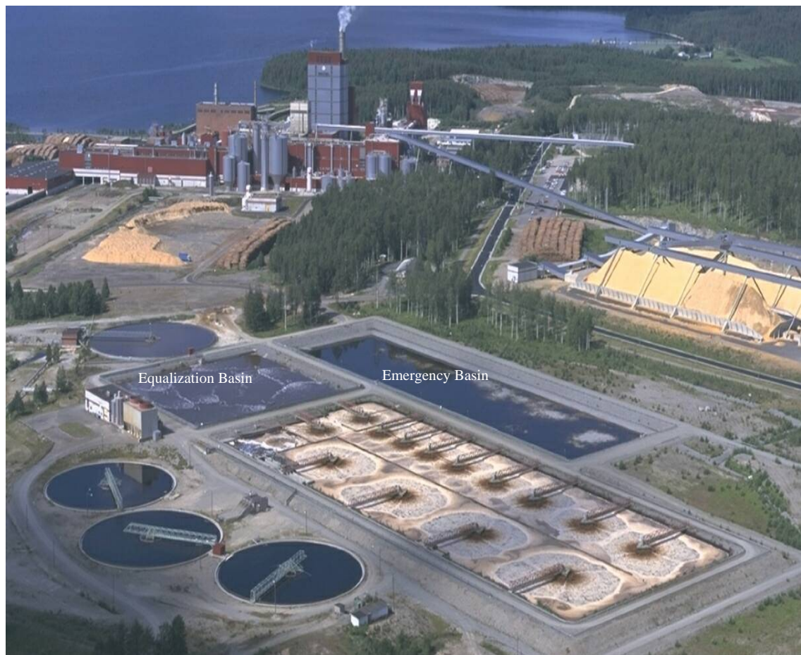
Figure 2/1. An Extended Aeration Activated Sludge Plant at a Pulp Mill in Finland
